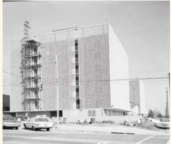
Construction of the Towers ("Honeycomb") residence hall, 1966
