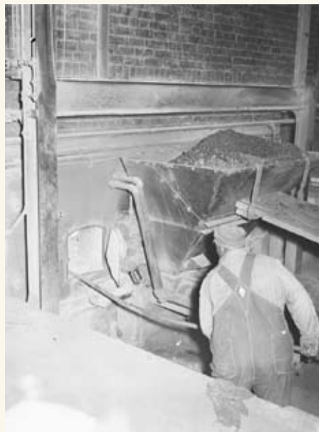
Coal-heating plant, 1940s
