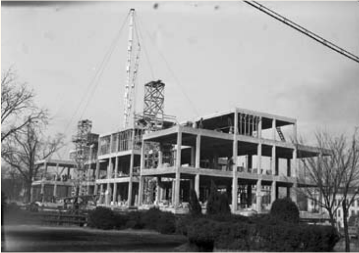
Construction of McKissick Library in 1939
