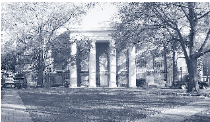
Installing new windows in the South Caroliniana Library.
