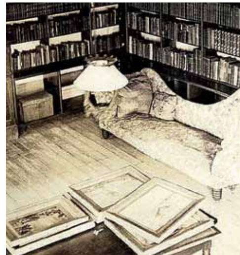
John Shaw Billings library at Redcliffe
