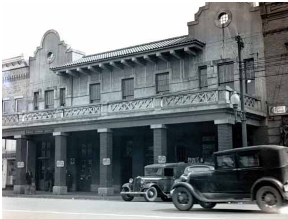
Union Station, Anderson, S.C.; architectural style unique to South Carolina
